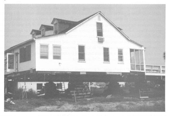
Figure 1. Photograph of a Pre-FIRM structure located on Sullivan's Island, South Carolina which was substantially damaged during Hurricane Hugo. NOTE: The structure has been repaired and is in the process of being elevated to or above the base flood elevation in accordance with NFIP requirements for substantial improvement (Refer to Question No. 9).
