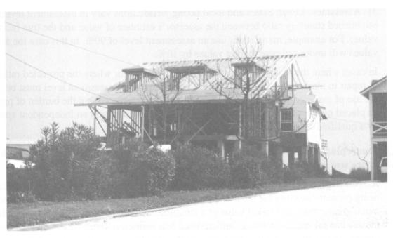
Figure 4. Photograph of a Pre-FIRM structure located on Folley Island, South Carolina which was damaged during Hurricane Hugo. NOTE: Both the damaged structure and the subsequent improvements (the adjoining addition) have been elevated to or above the base flood elevation in accordance with NFIP requirements (Refer to Question No. 24).
