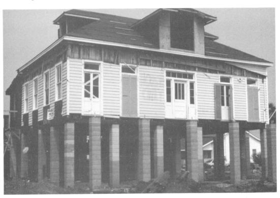
Figure 3. Photograph of a Pre-FIRM structure located on Sullivan's Island, South Carolina which was substantially damaged during Hurricane Hugo. NOTE: The structure is in the process of being repaired and has been elevated to or above the base flood elevation in accordance with NFIP requirements (Refer to Question No. 14).
